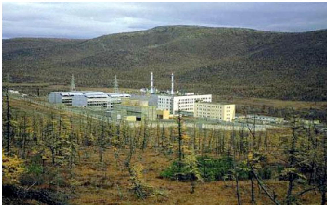
▲ Bilibino Nuclear power plant
