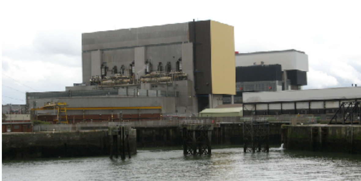
▲ Heysham Nuclear power station
