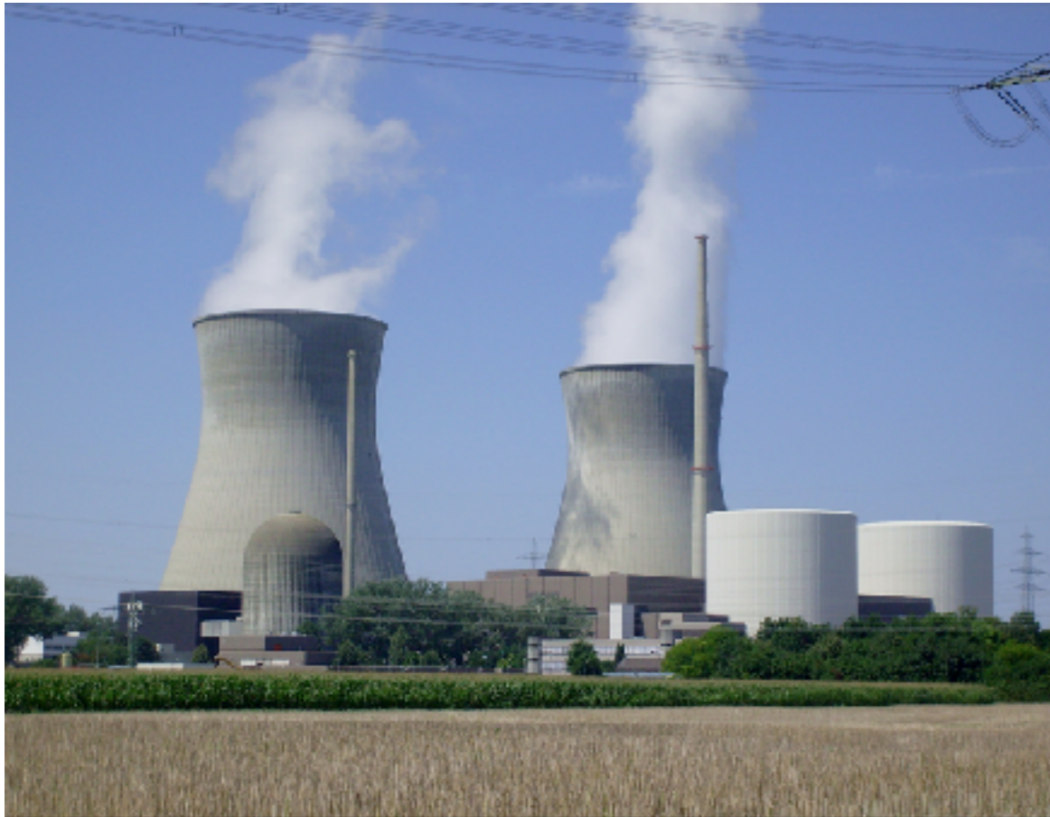
▲ Gundremmingen Nuclear power plant
